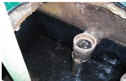
Root Clogged distribution box on a 4-year old system
