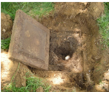
Root Clogged distribution box on a 4-year old system
