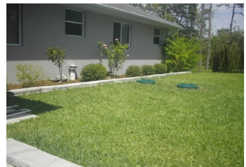
Excavations are restored .
